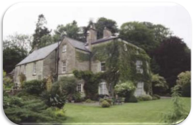
Cowley Old Rectory, June 2005 iii
